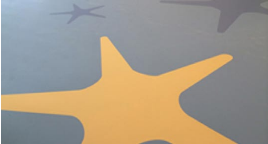
Resilient floor installation by AFR: Manhattan Star Academy
